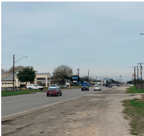
South Roosevelt Avenue facing North
