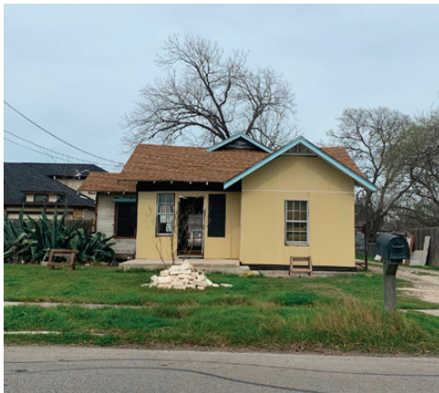
A Single Family home being renovated in the plan area.
